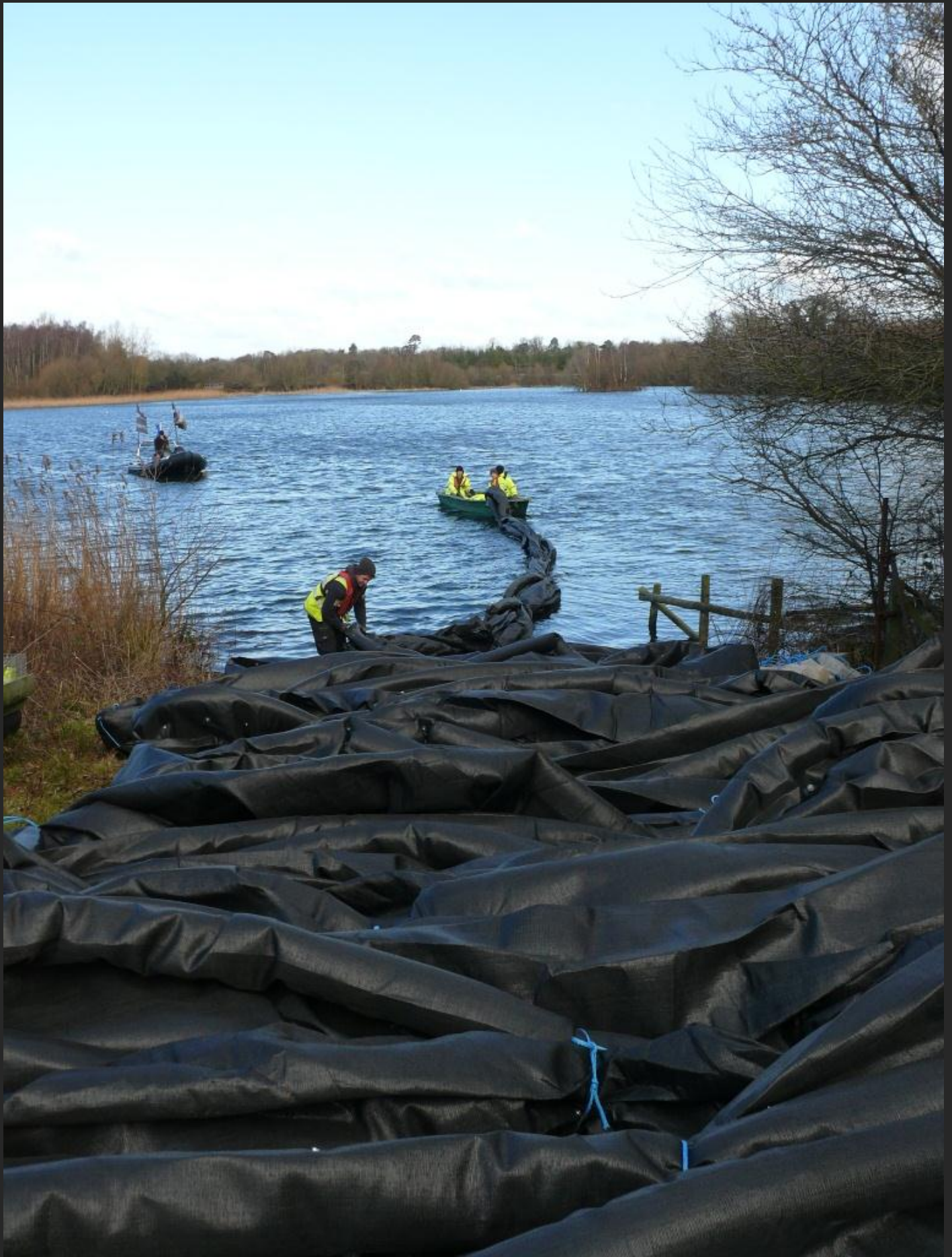
Once the netting team had cleared the area of fish the 160m fish exclusion curtain was floated into place, the dive team were on standby ready to deploy the anchors required to hold it where deployed for the period of the trial which could be several years.
