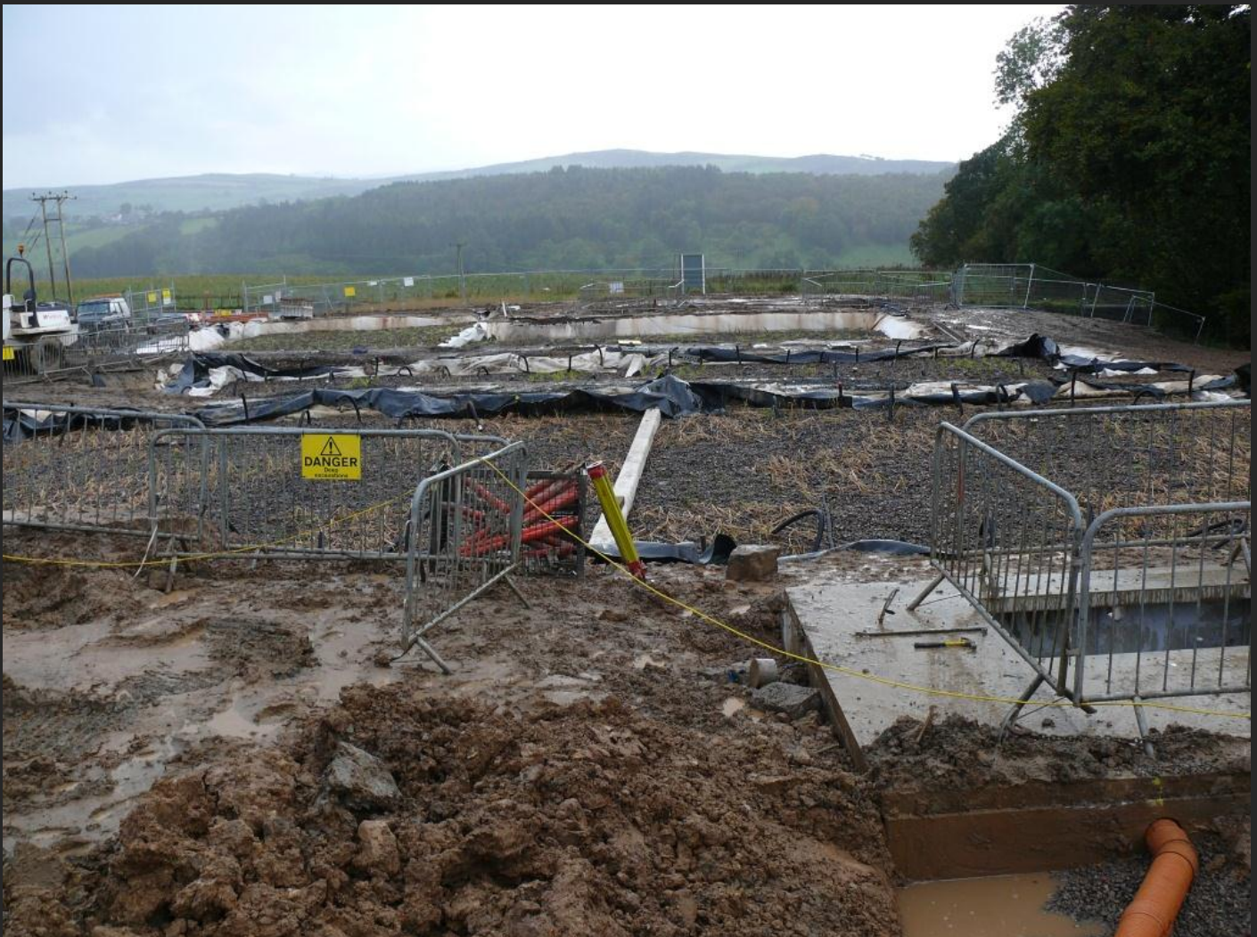
Cartland well underway when AquaticEngineering arrived on site in October 2012
